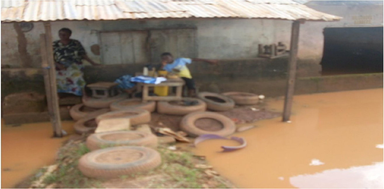
Figure 13. Raised walkway with old vehicle tires as a strategy for reducing erodibility.
