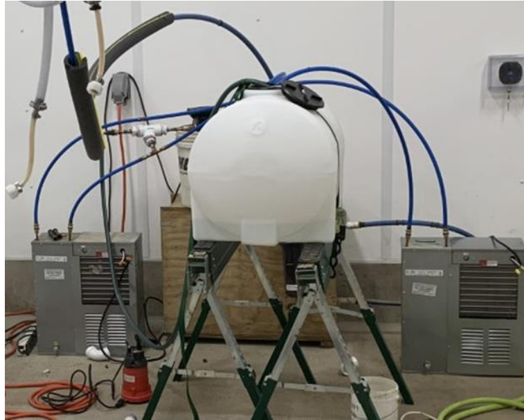
Figure 14: Coolant reservoir on elevated stand beside the water chillers and in front of the supercharging pump in an unsuccessful preliminary design configuration of the coolant recirculation system at USDA-ARS Farm Animal Behavior and Well-Being Laboratory (FABL) animal holding room.
