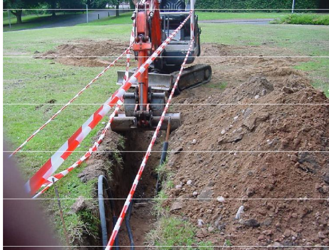
Figure 20. A photograph of a laying ground-loop heat exchanger (Abdeen Mustafa Omer, 2009).
