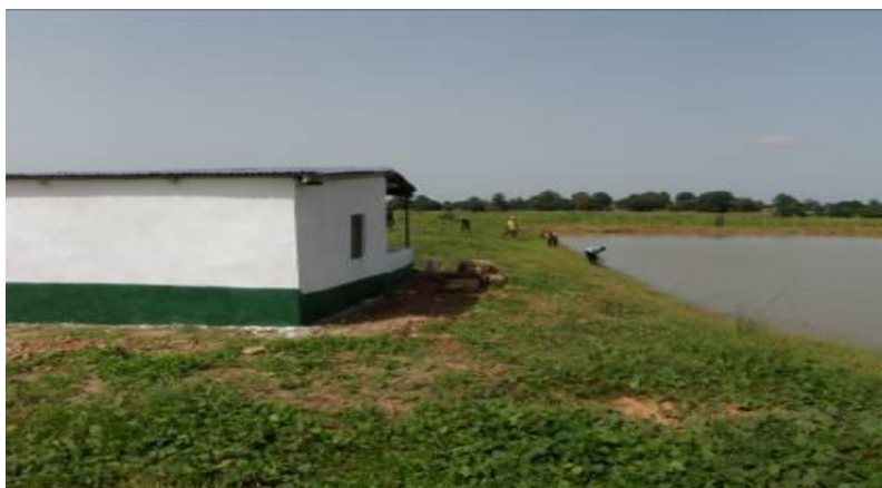
Figure 3. FBO managed fish pond at Golinga irrigation scheme (GIP).
