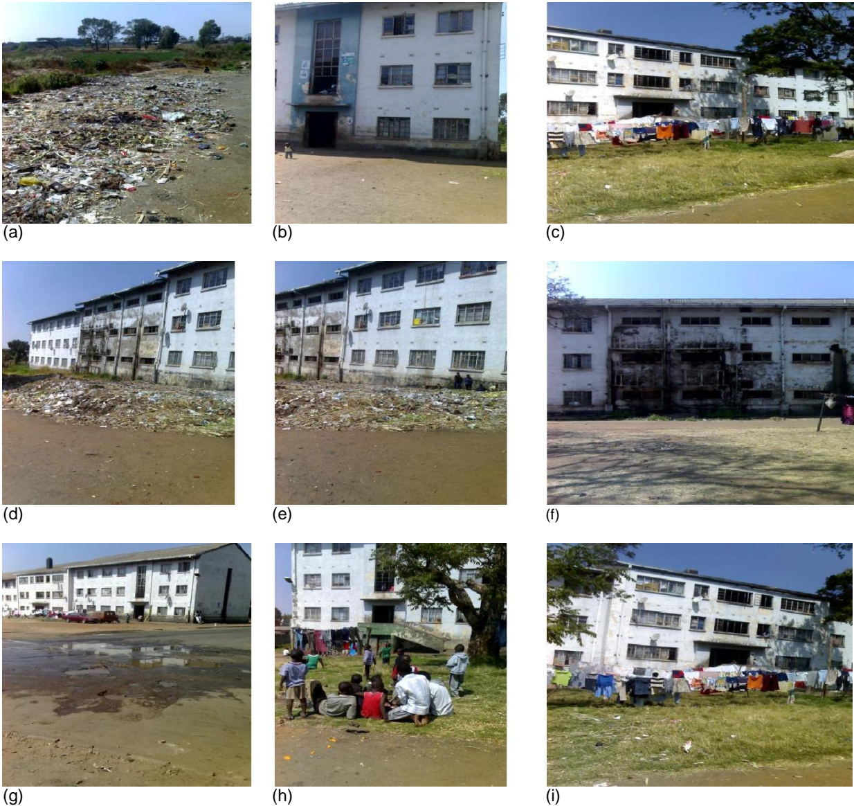
Figure 4. Matapi Habitat, Hostel Buildings and Lifestyle of the Dwellers in 2008. (a) An informal dumpsite in Matapi area. A child is seen sitting on the dump. (b) A child at the entrance of one of the hostel blocks. The hostel is in a messy state. (c) Hostel dwellers use washing lines in commonality. Cases of stolen clothes are many. (d) Another dumpsite just behind hostel block. The ablution area of the block is the worst vandalized. The responsible authorities (City of Harare) has cited financial and fuel problems for failure to discharge the waste collection service. (e) Children play on the dumpsite. See satellite antennae hanging on the walls. The dwellers may be poor in other respects but they thrive to be information-rich. But what is also the challenge of the media. (f) A building in a worst state of deterioration. As residents share the communal ablutions, they quarrel, gossip, preach the gospel one to another and share the latest news. What an admixture of activity and involvement! (g) See the parked cars and the road - full of potholes with water. (h) A less child-friendly environment (i) Compare with (c).
