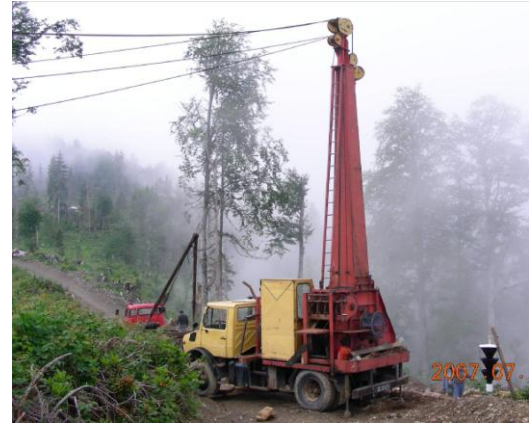
Figure 1. Urus Mill cable crane in felling area.
