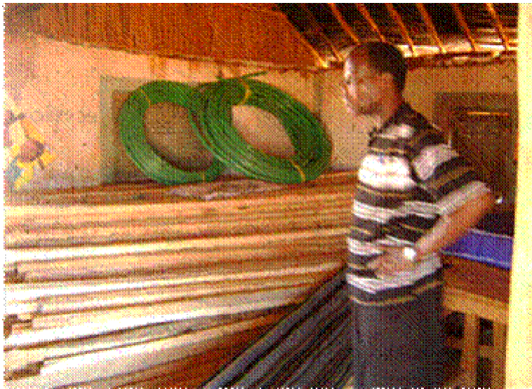
Figure 2. PVC pipes, Wood and metal bars (Materials for fabrication of cages and walkway)
