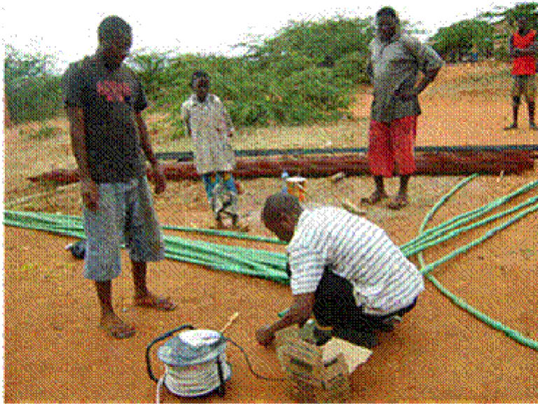
Figure 4. A Technician melting a pvc pipe to fix during fabrication of cages
