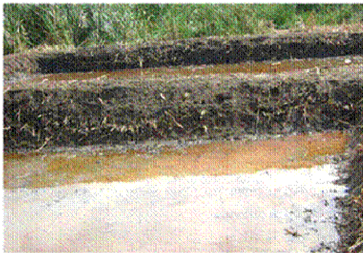
Figure 14. Two of the six ponds excavated being compacted and partly filled with water
