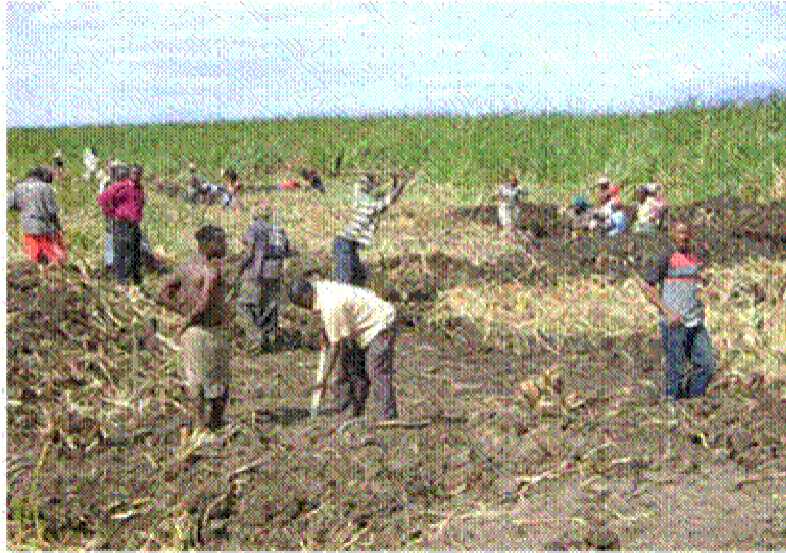
Figure 11. Community members engaged in ponds excavation adjacent to Lake Jipe
