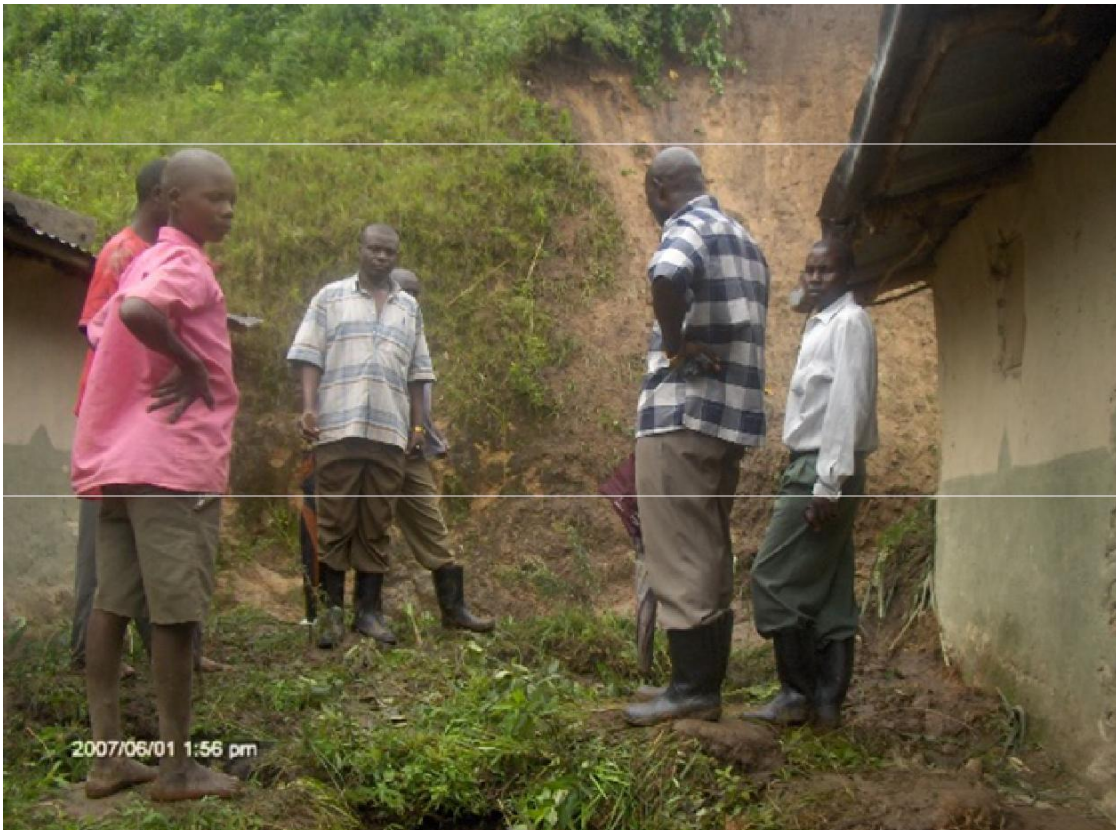
Figure 10 A. Landslide due to house construction. Two children were killed in 2007.
