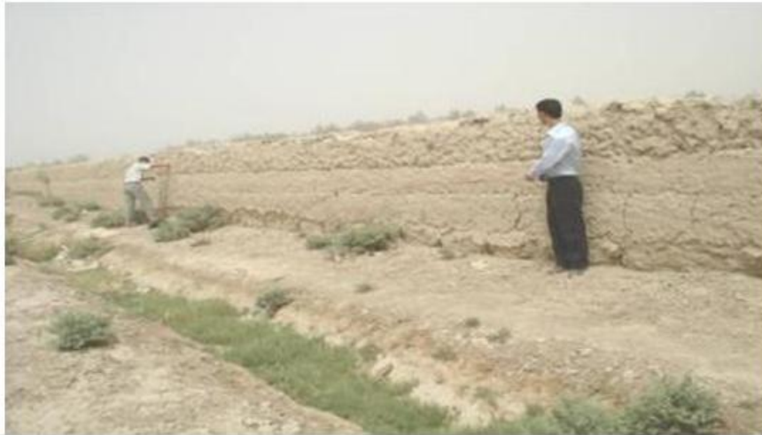
Figure 2. View of Mud wall wind break which used in this study as an abiotic windbreak
