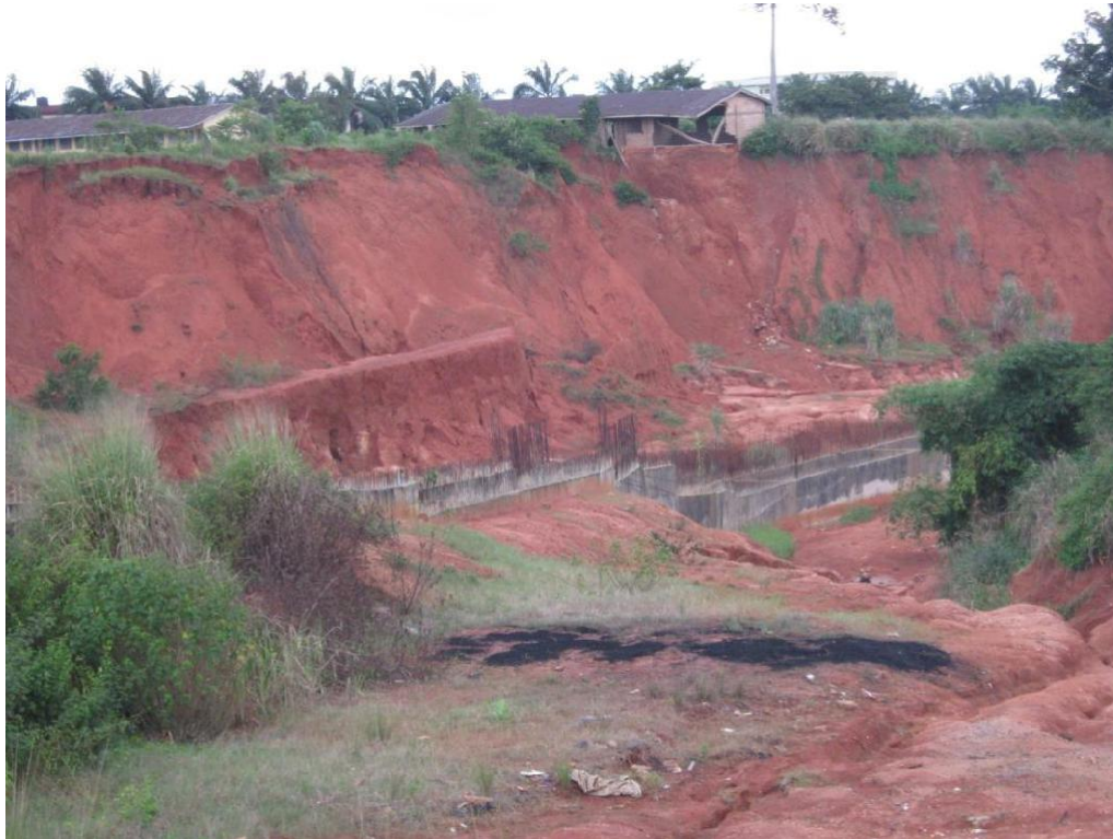
Plate 1. Ogbesan Gully, Benin City showing school building caving in and the failed community effort of drain construction to solve the gully problem.
